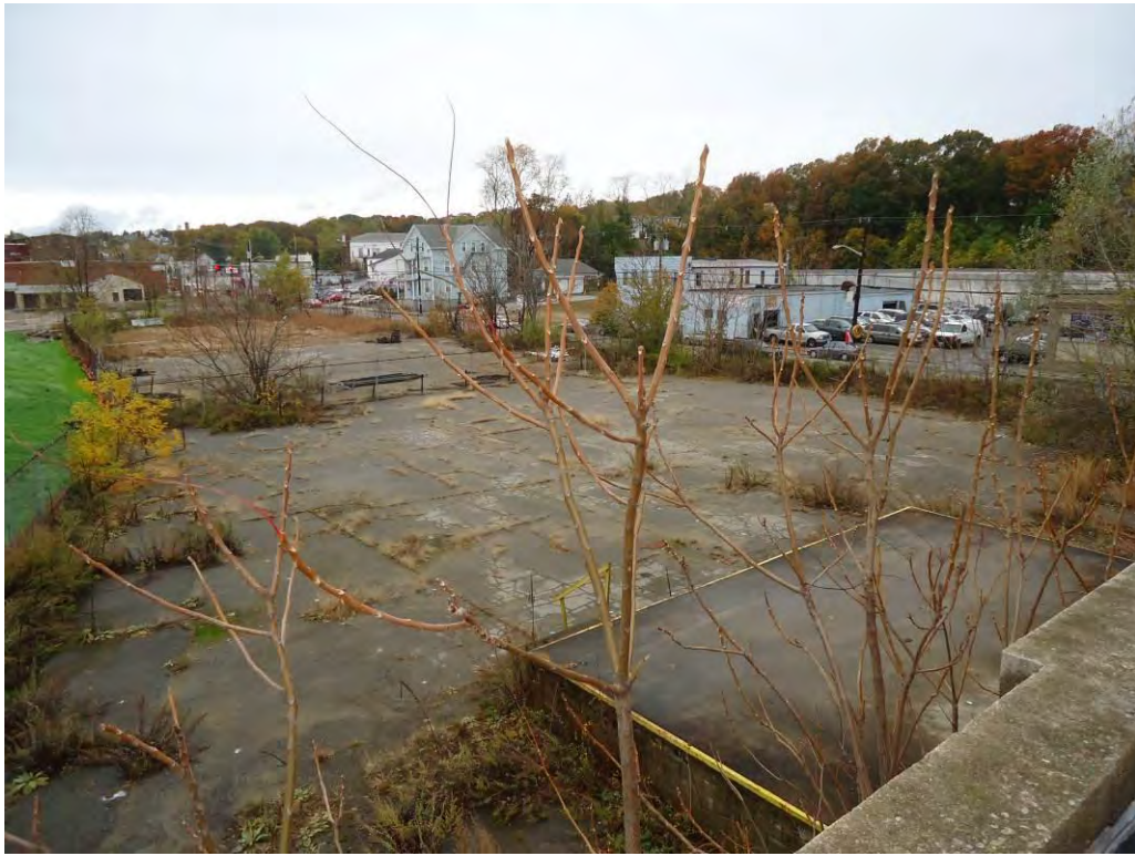
Photograph 9: Site grounds, looking west from the roof of the subject-site building.
