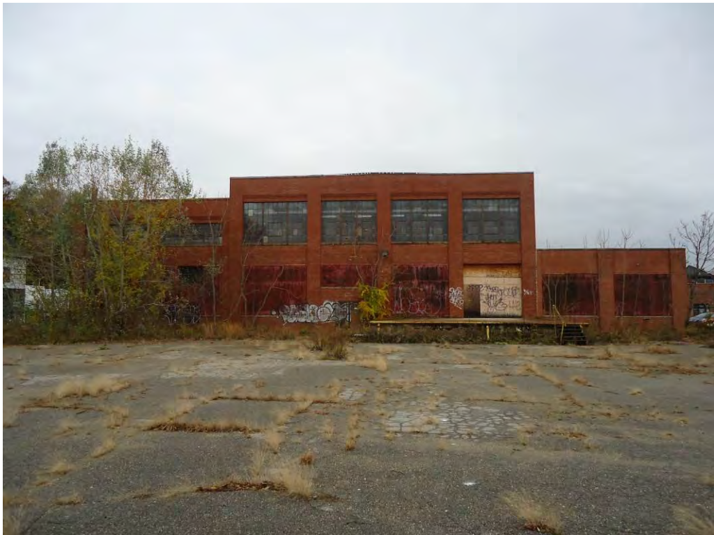
Photograph 8: West side of the site building
