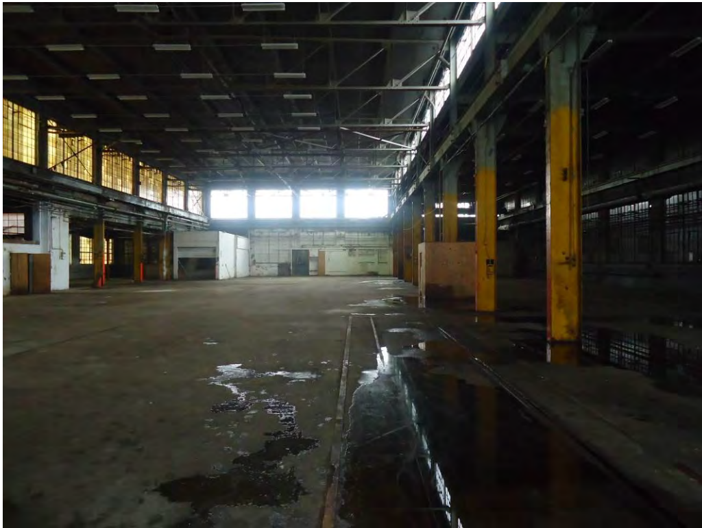
Photograph 1: Site building looking west
