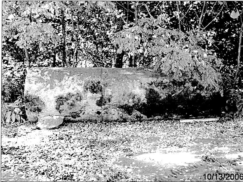
Photograph 1. Looking in a westerly direction at Lot 430. A view along the bottom of the 2,000 gallon #2 fuel oil UST.
