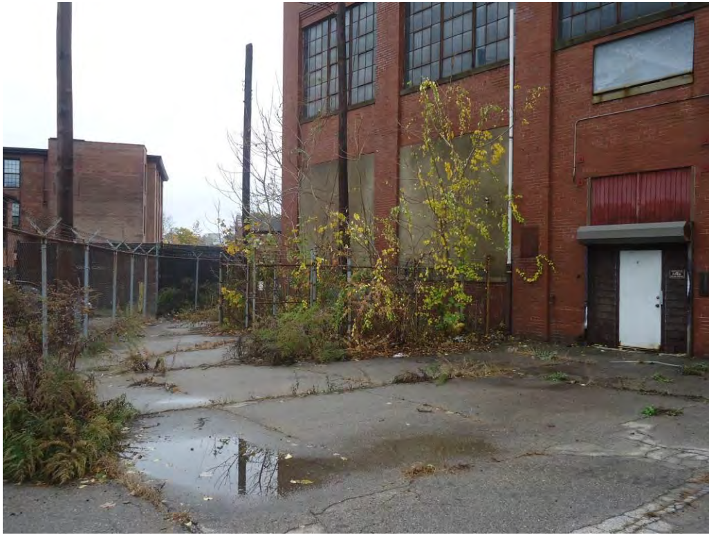
Photograph 11: Former transformer area (center)
